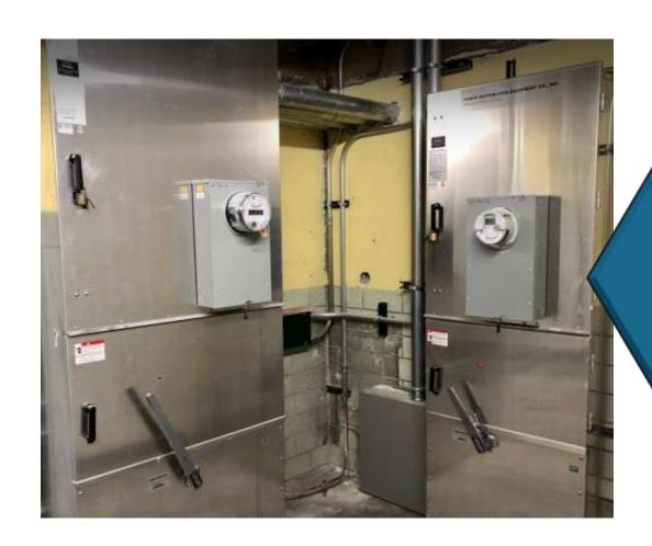
Installation of 1) entirely new electrical panel room off the social hall 2) upgraded electrical wiring to the north end of the building and 3) a new ComEd transformer in the alley to accommodate our increased electrical needs.
