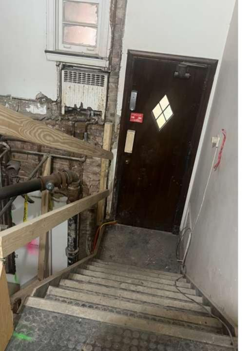
Half of the existing north stairwell was retained, while the other half had to be relocated/ newly-constructed to make room for the elevator and lobby.
