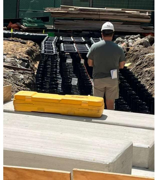
Trenches with eco-friendly water retention systems were installed for the six courtyard trees.
